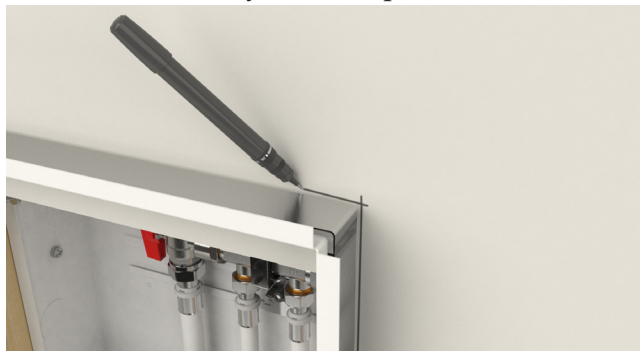
Mark the outside of the frame on the plaster board
